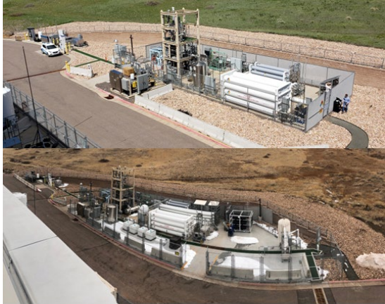
NREL HITRF Station Expansion Under IHS Project
